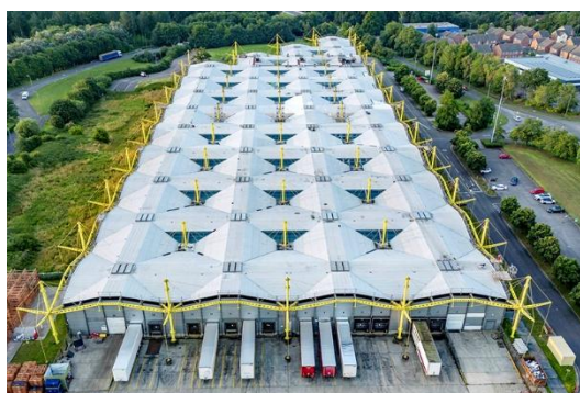
25,000m 2 – refurbishment – substrate retained
